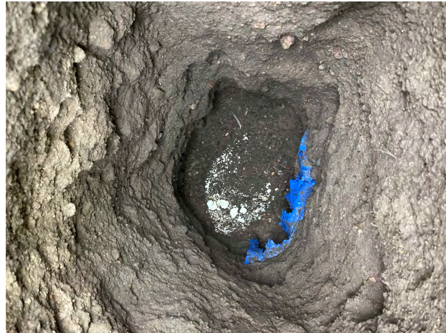
104 PHOTO OF C3D POINT #6 (POTHOLE 7) SU06
