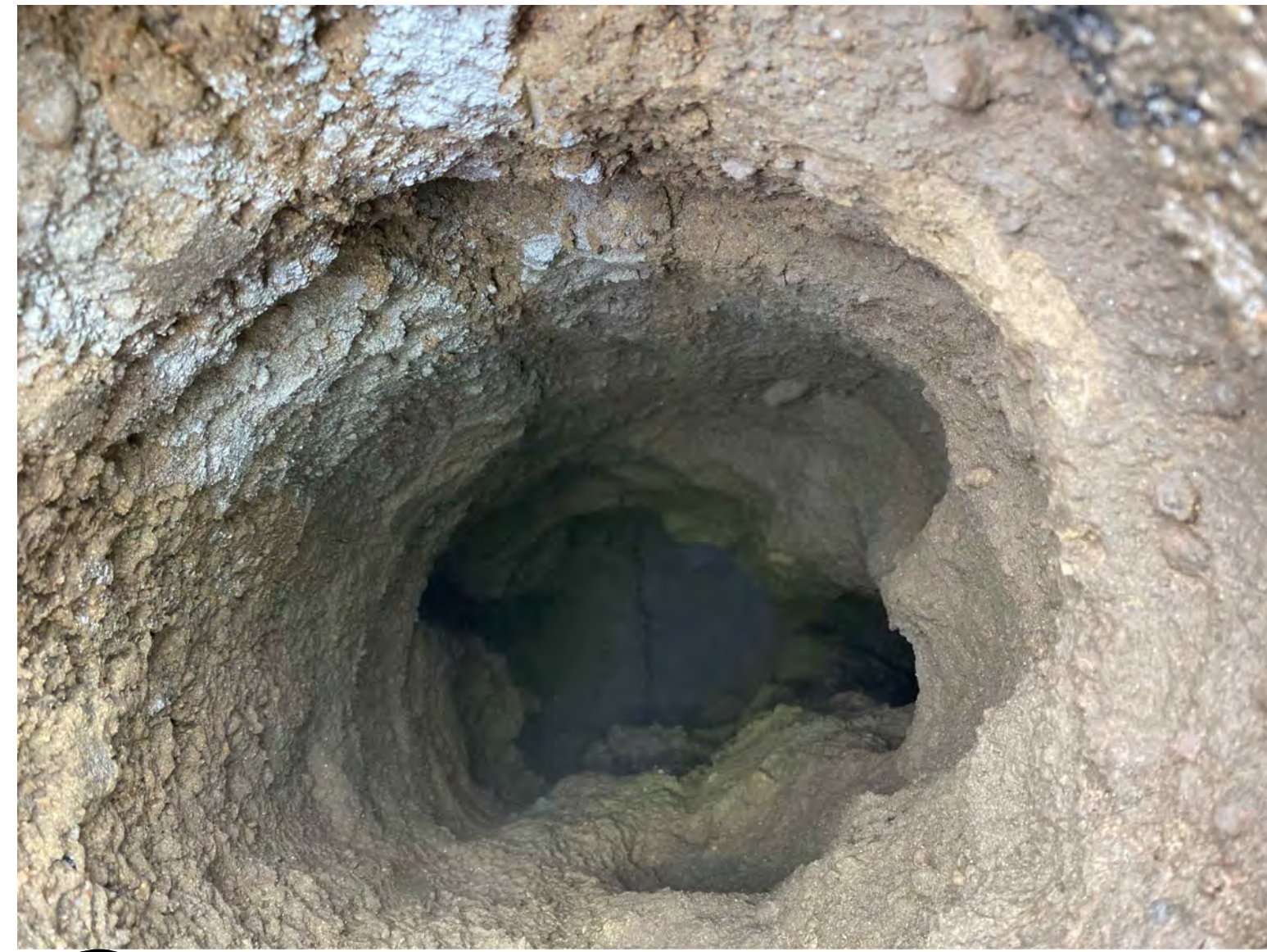
102 PHOTO OF C3D POINT #4 (POTHOLE 4) SU06
