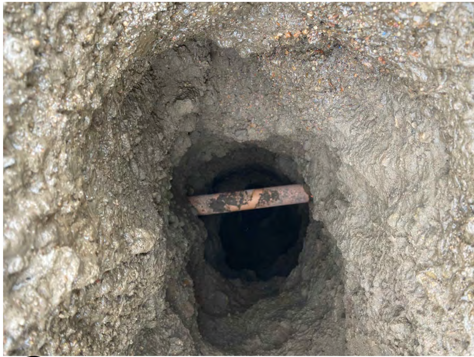
109 PHOTO OF C3D POINT #11 (POTHOLE 11) SU07
