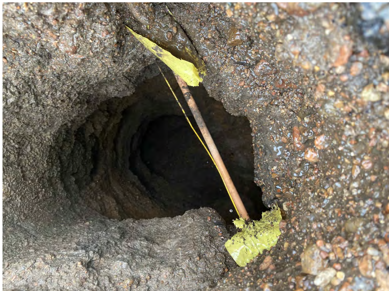
106 PHOTO OF C3D POINT #8 (POTHOLE 10) SU06
