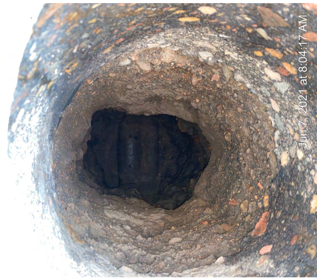
111 PHOTO OF C3D POINT #13 & #14 (POTHOLE 13) SU07
