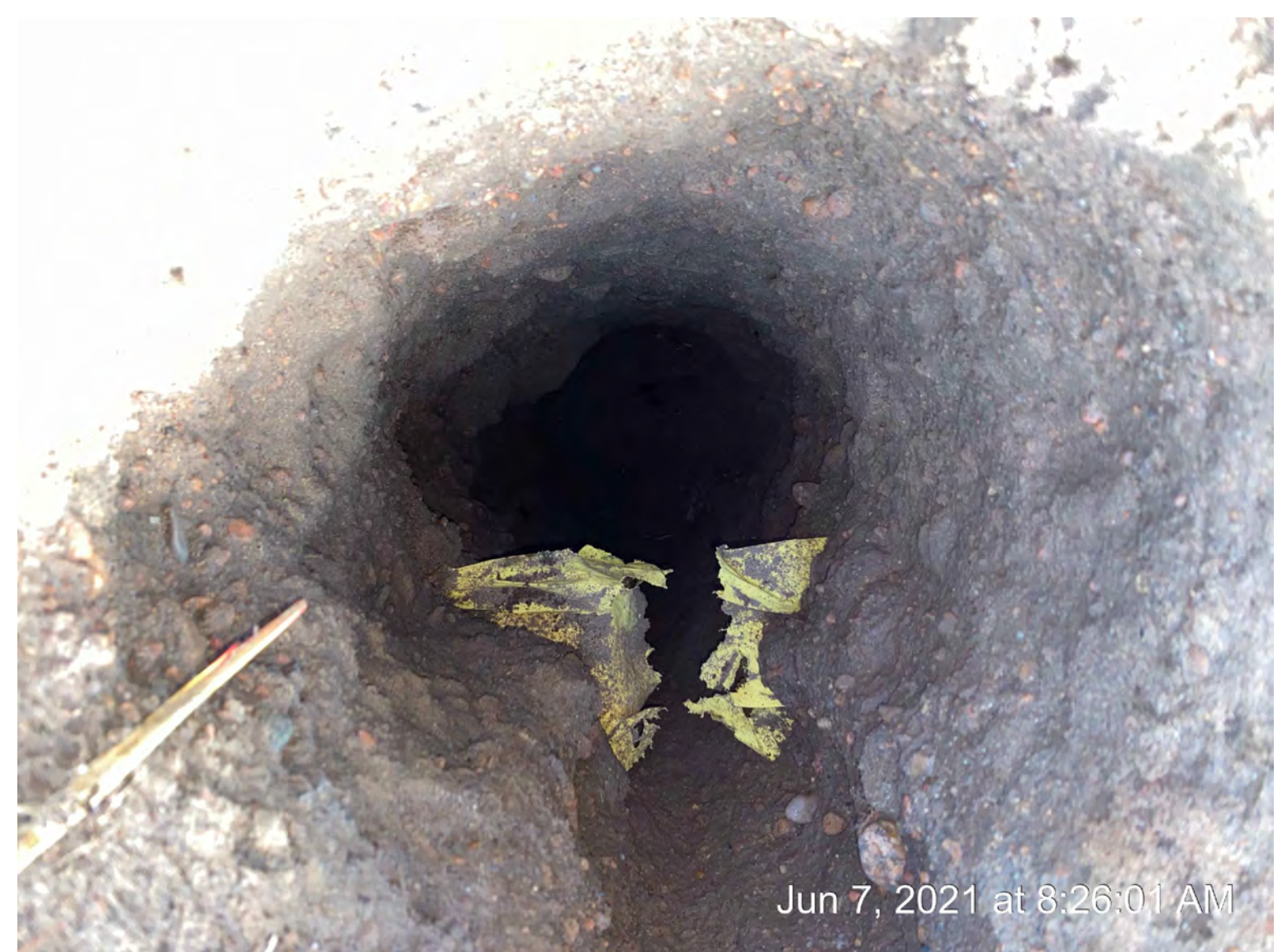
108 PHOTO OF C3D POINT #10 (POTHOLE 10.2) SU06
