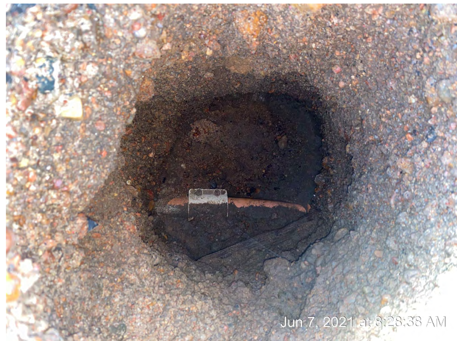
107 PHOTO OF C3D POINT #9 (POTHOLE 10.1) SU06
