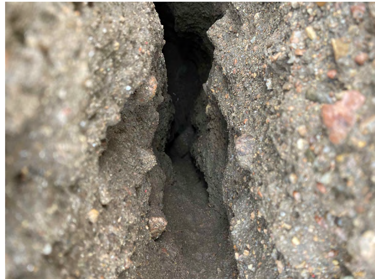
105 PHOTO OF C3D POINT #7 (POTHOLE 8) SU06
