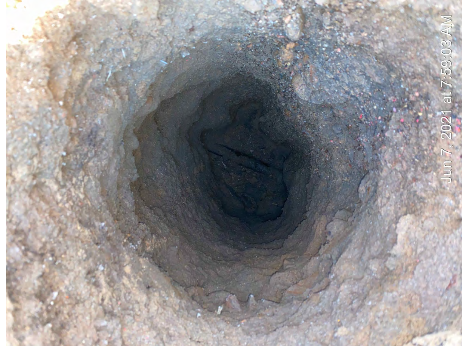
113 PHOTO OF C3D POINT #16 (POTHOLE 15) SU07
