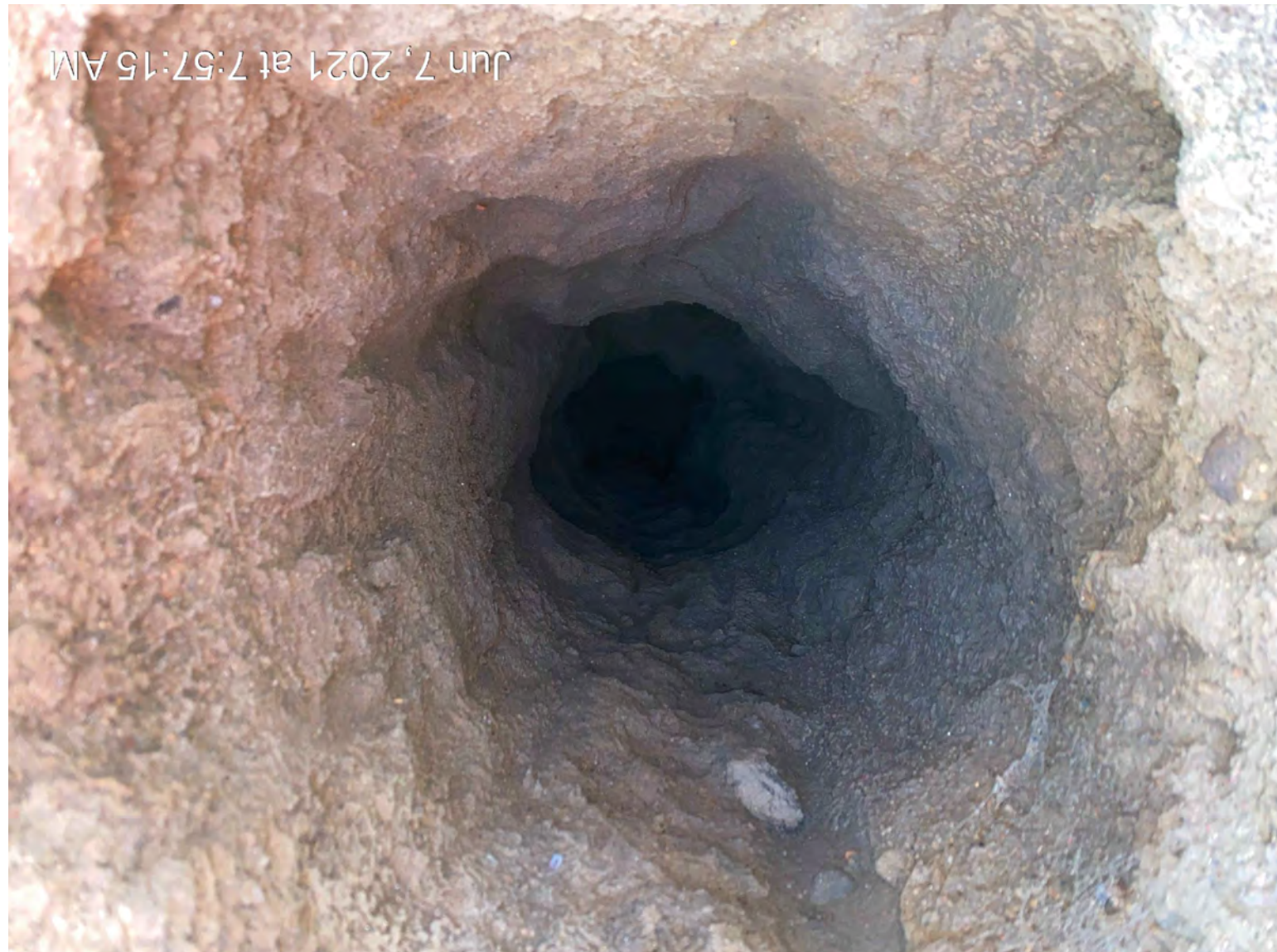
112 PHOTO OF C3D POINT #15 (POTHOLE 14) SU07
