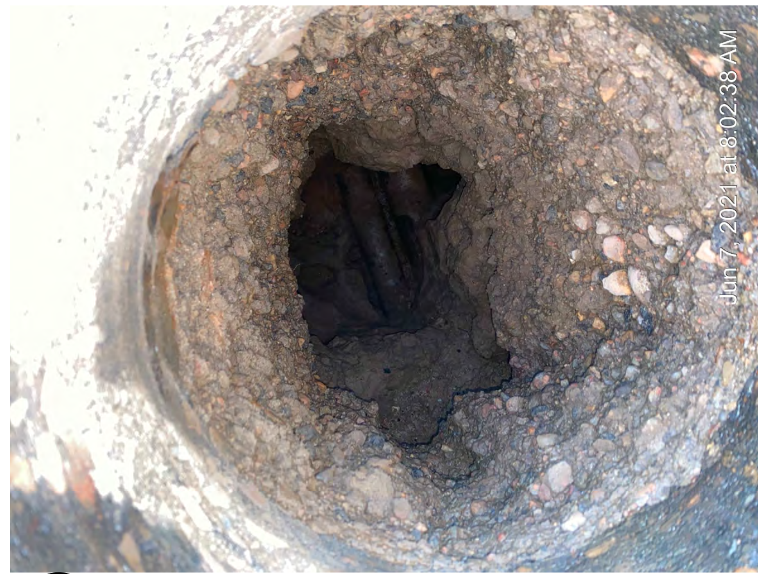
110 PHOTO OF C3D POINT #12 (POTHOLE 12) SU07
