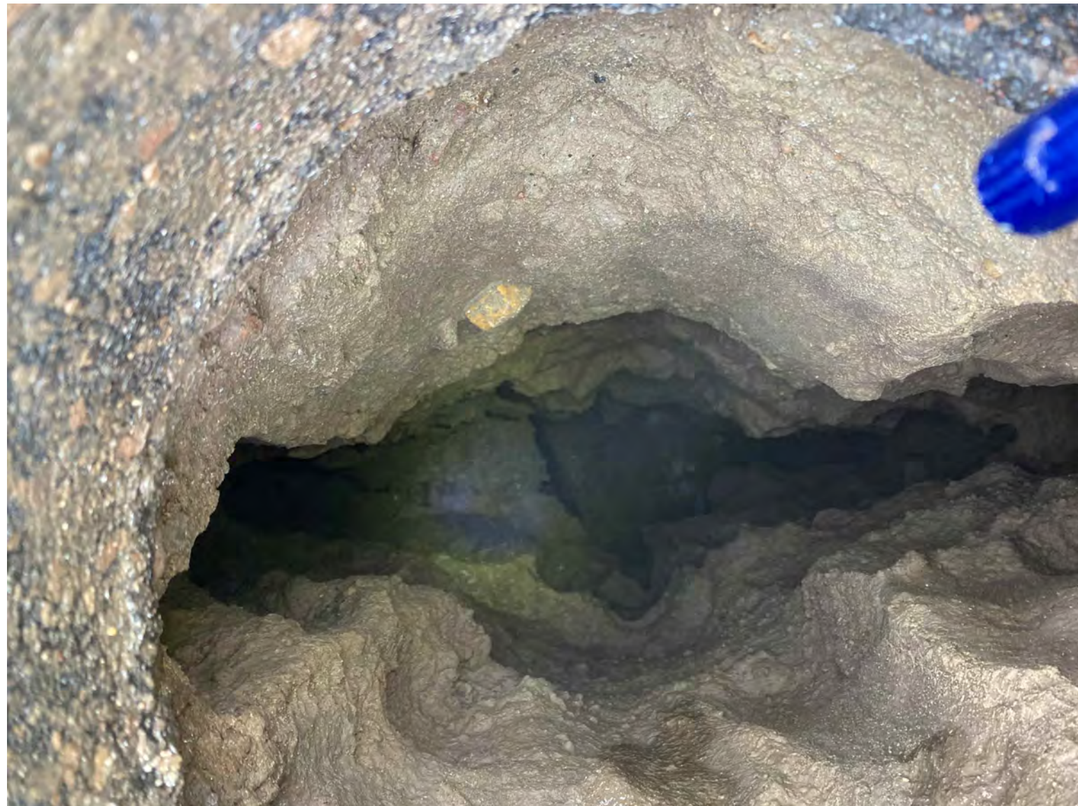
103 PHOTO OF C3D POINT #5 (POTHOLE 6) SU06
