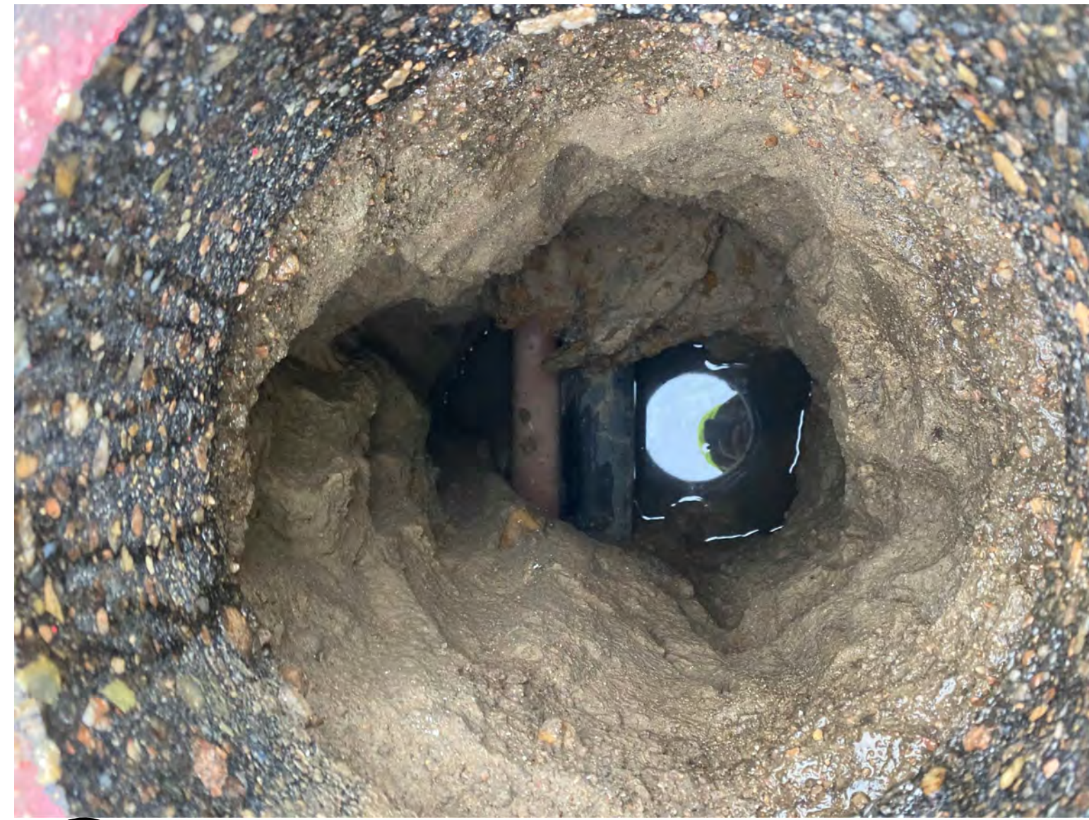
101 PHOTO OF C3D POINT #3 (POTHOLE 2) SU06
